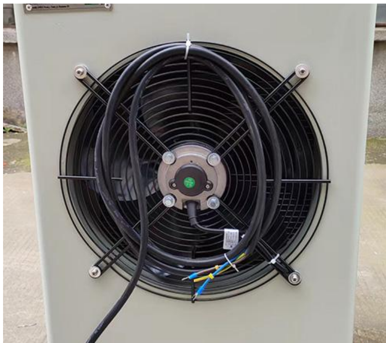
Aluminum fin+fan Condenser
